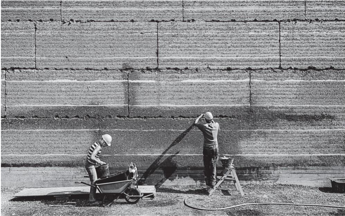
Figure 13: Filling and retouching the joints 86
